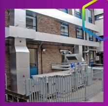
**Continued from page one** The project included DI water, process chilled water, process extract as well as small power and data fitted in dado trunking. Air conditioning was mounted externally and consisted of an air handling unit, chiller, chilled water pipework, LPHW pipework from the university's existing system, humidifiers and controls to achieve the designed close control criteria.
