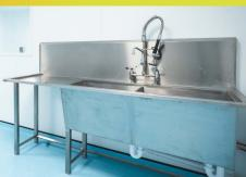
Hot and cold water supply can be installed to handwash and utility sinks as well as process equipment that may have a demand. Drainage can be accommodated either via pump or gulleys – for Pharmaceutical applications 316 stainless steel drainage and traps can be provided.
