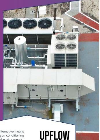
A popular alternative means of providing air conditioning to controlled environments is by using smaller package upflow/downflow units either directly ducted to Fan Filter Units (FFUs) or ducted to a plenum where FFUs draw a common supply.
