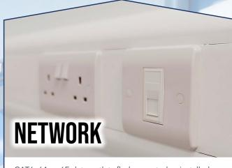
CAT6, 6A or 6E data outlets flush mounted or installed within trunking, cabled back to network patch panel for client connection to host building server. Can also be incorporated into the EMS and BMS.
