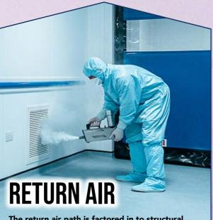
The return air path is factored in to structural components, either via bespoke panels with hollowed channels to accommodate sufficient airflow or as columns produced from the same materials used for wall construction. These columns can also be used as service chases to conceal process and plant utilities.
