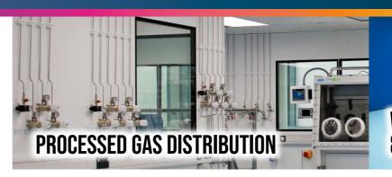
Highly filtered compressed air can be provided with compressors, filtration, transair pipework and a range of fittings for process requirements. In addition, a vast range of gasses, either from cylinder or generator, can be integrated into the facility design with appropriate pipework, valves and manual or digital control systems with appropriate alarms where required.
