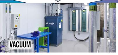
House vacuum for cleaning activities can be provided via a centralised vacuum system. This enables a number of rooms to have a wall-mounted connection to a central pump that is housed externally to the controlled environment with filtered exhaust. Vacuum pumps and pipework can also be provided for process applications.
